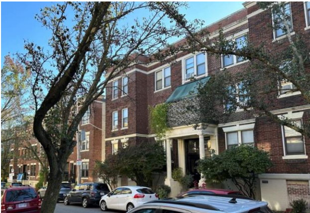
The Allston Brighton Community Development Corporation will retrofit and decarbonize 33 apartments on Carol Avenue in Brighton. (Courtesy of the Allston Brighton Community Development Corporation)
